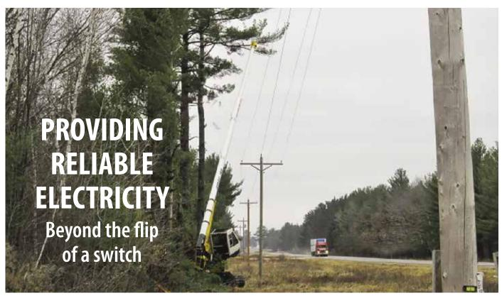
lark Electric Cooperative has numerous maintenance programs that help provide safe, reliable electricity. One of the most important programs the cooperative performs is our vegetation management program. This program is twofold. First, trees are cut and trimmed from within the right-of-way. Once the trimming and clearing process has been completed, a herbicide application is applied to help reduce regrowth within the right-of-way.
